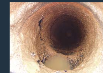
Pipeline before cleaning by Pigtek
